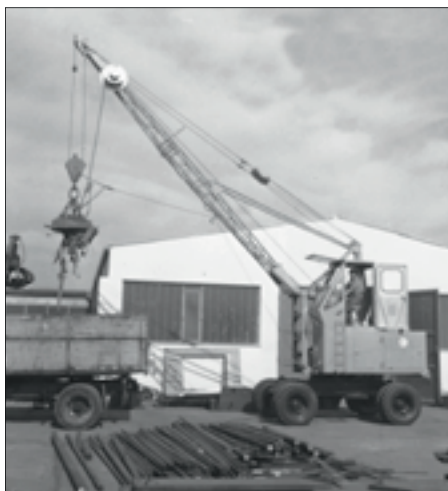
1962: rope-driven S833 with elevated operator cab
