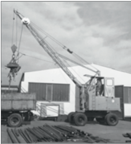
1962: rope-driven S833 with elevated operator cab
